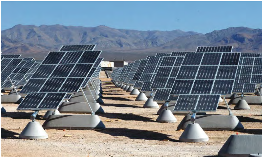
Figure 3. One-axis tracking solar power plant
