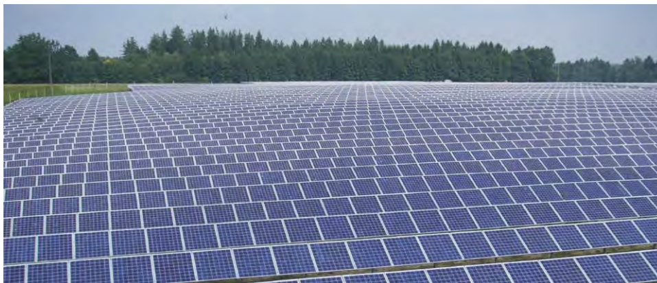
Figure 2. Fixed PV solar plant
