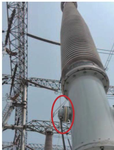
Figure 11: Insulation of the live display device of the 5062C-2 Knife Gate gas chamber
